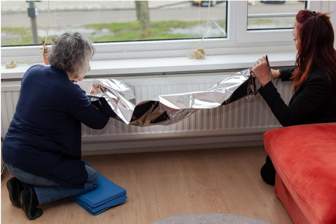
Figure 16: Installing radiator foil in a resident's home (by Nanna van Hout - JMA)
